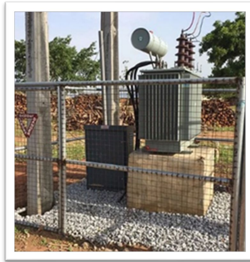
Figure 1. Typical distribution transformer used for rural electricity distribution
