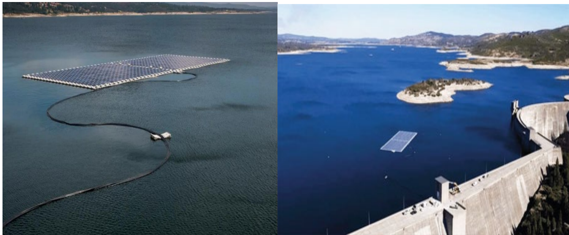
Figure 2: World's first hybrid hydro and floating solar plant at Alto Rabagão [3]
