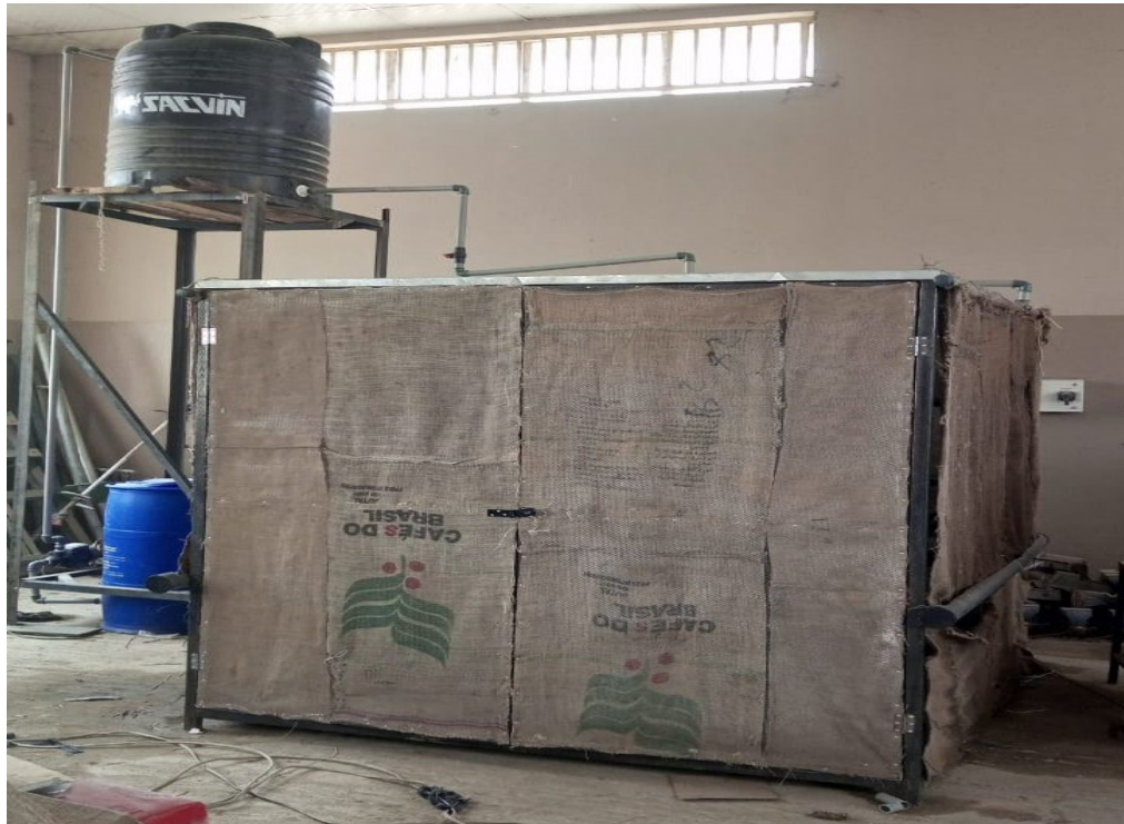
Plate 1: Photograph of the completed evaporative cooler framework
